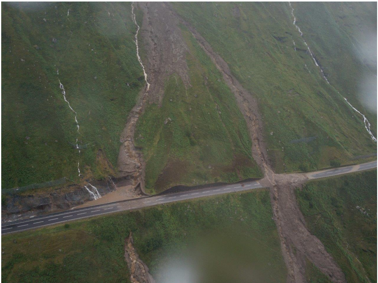
A permanent solution is needed for the A83 Rest and Be Thankful © BEAR
